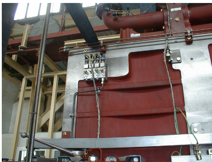
Built-on group of lubricating oil pressure sensors 1106 and 1104
